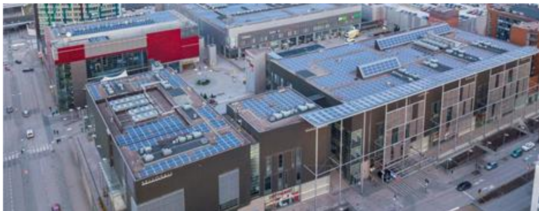
Figure 5. PV Panels on Sello Centre. Source: Siemens
