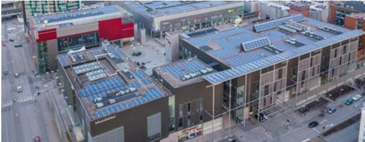
Figure 12. PV Panels on Sello Center. (Source: Siemens)
