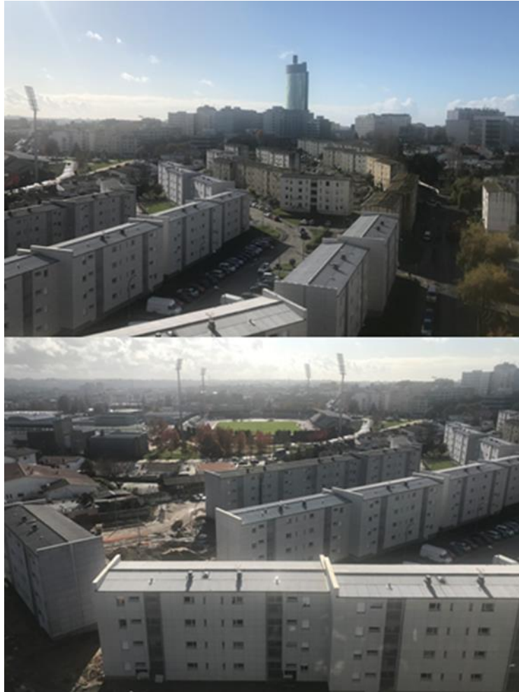
Figure 26: Sobreiro District - Refurbishment Project ongoing under PARU- Maia (Own elaboration)
