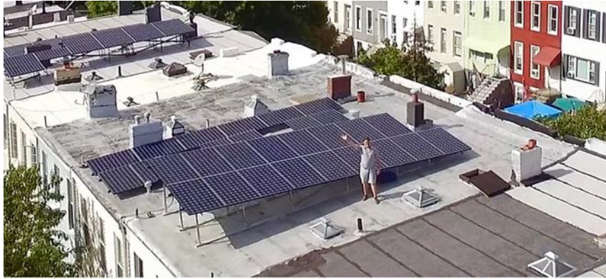
Figure 10: Solar rooftop panels in Brooklyn [22]
