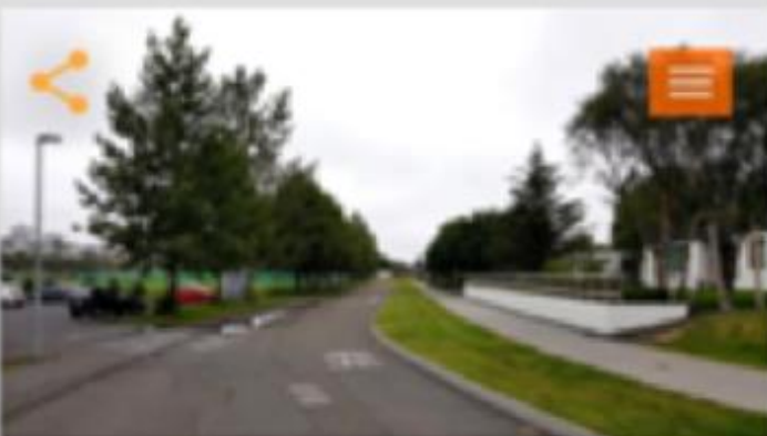
Repairing holes on Traðarland
