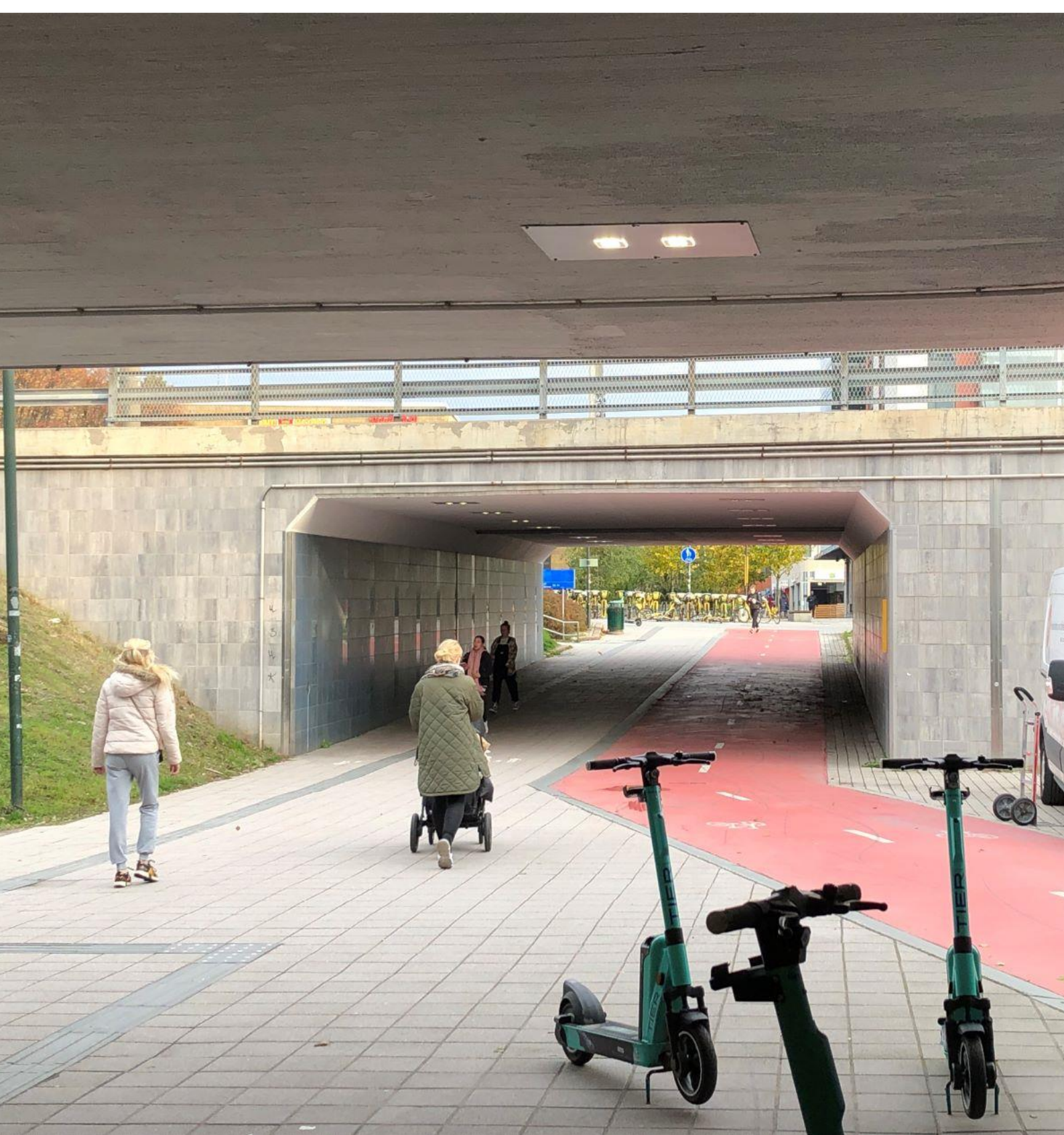
Figure 2. Pedestrian bicyclist underpasses at the Leppävaara station area. A dedicated bicycle path next to the pedestrian path runs under the train tracks (front) and the adjacent motorway (back). Electric kick scooters parked (free-floating system) next to the stairways leading up to the train platforms. Photo: author.
