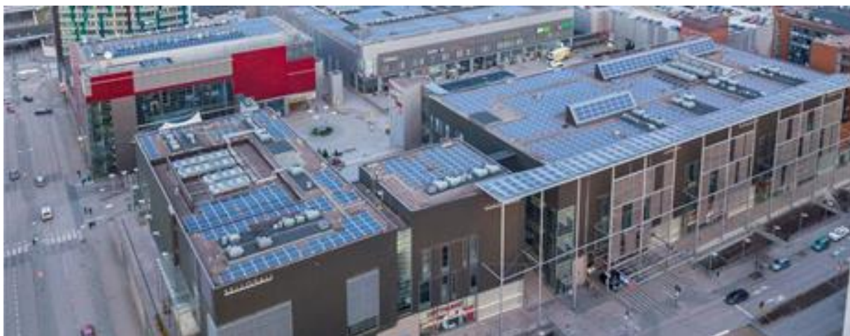
Figure 4 PV Panels on Sello Center. (Source: Siemens)
