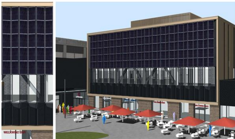
Figure 4. Lippulaiva will have extensive amount of onsite energy production: Sketch of solar panels in Lippulaiva façade.
