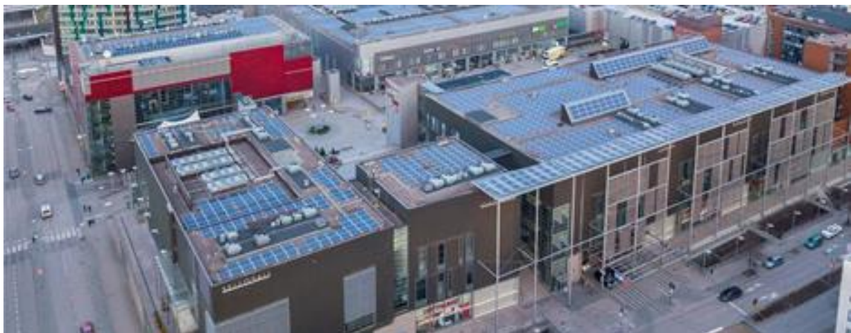
Figure 6 PV Panels on Sello Center. (Source: Siemens)
